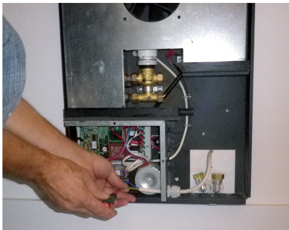
Picture No 5 - Electrical connection of the rough
